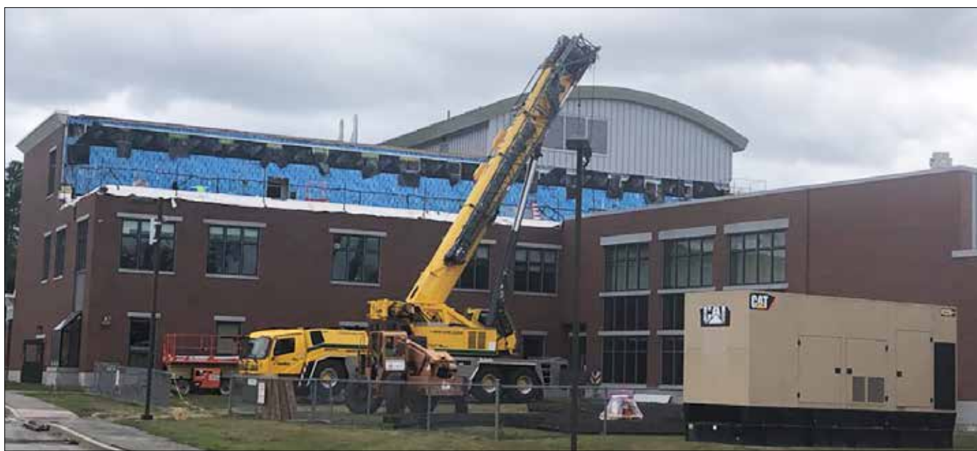
CONSTRUCTION WORK IS ON SCHEDULE for the 3rd floor build-out at Hampden Academy, according to Director of Facilities Bill Booth. The crane arrived on site August 10, and the steel was lifted into position after about a week. The next items needed are the windows, which have been delayed—not because of the steel framing but because of the glass. Mr. Booth said he still expected the project to be completed by April. He said there should be minimal disruption to the students. There may be some background noise when the construction crews install the framing and shoot it down into the concrete deck. Also, the third floor corridor will be partitioned to ensure that the construction workers can get up to the project area, and the stairwell closest to the football field will be off limits except for emergency egress.
